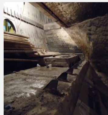
Partial re-lining of a grate combustion chamber.
